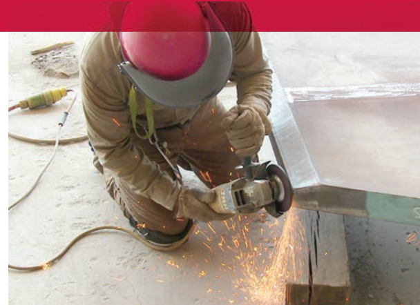
Grinding on a platform for weld preparation.
