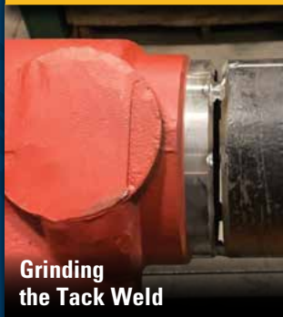
Root Pass Grinding
