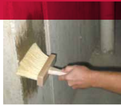
Applying waterproofing material with a masonry brush.
