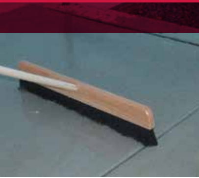
Creating texture on newly poured concrete with a cement finishing brush.
