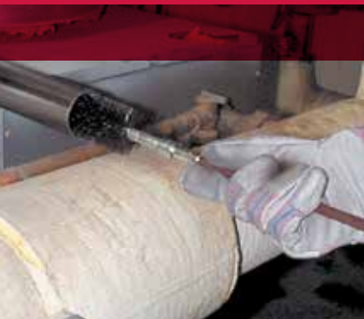
Cleaning boiler pipes with a flue brush.
