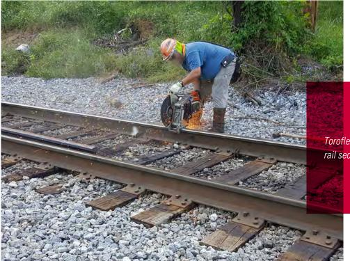
Toroflex PRO wheel cutting a rail section for repair.
